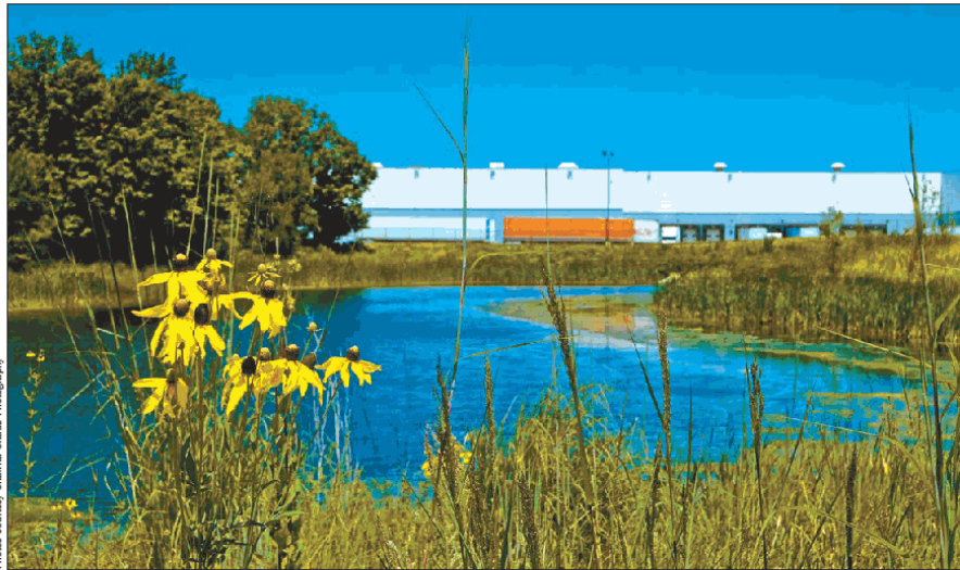
Warehouses and distribution centers go hand and hand with nature at AmeriPlex.
