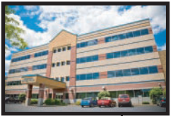
1st joint venture, Memorial Skyway Plaza, completed; South Bend, IN- 1989
